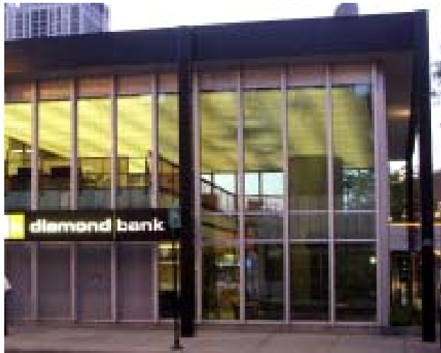
Glass curtain walls and a luminous ceiling make the interior of the bank readily visible from street. Instead of security, bank architecture emphasized transparency and customer service in the post-World War II period.
